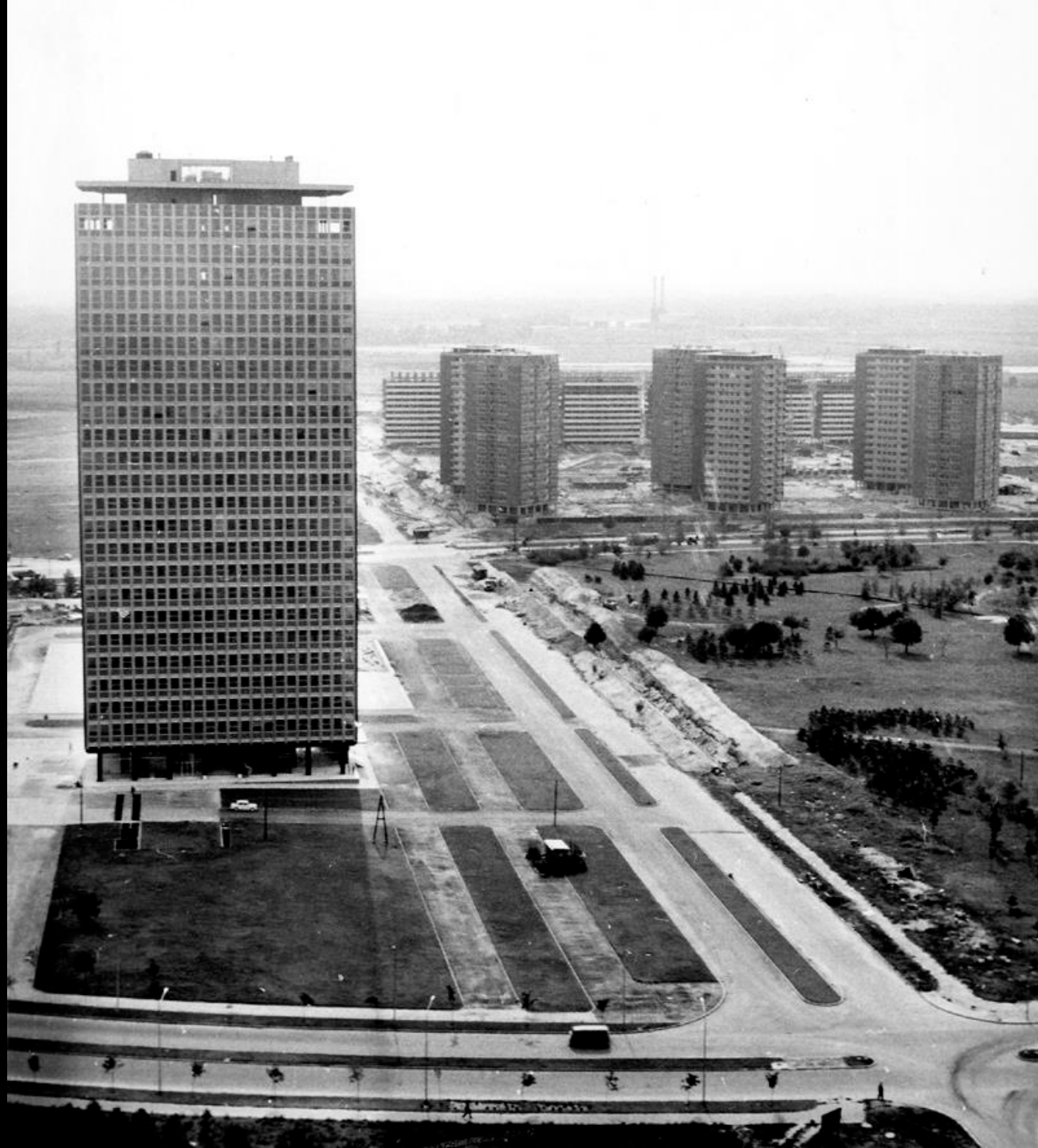
Headquarters of the League of Communists of Yugoslavia and mass housing in the neighborhood unit Block 21.
