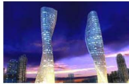
Central business district de Guangzhou
