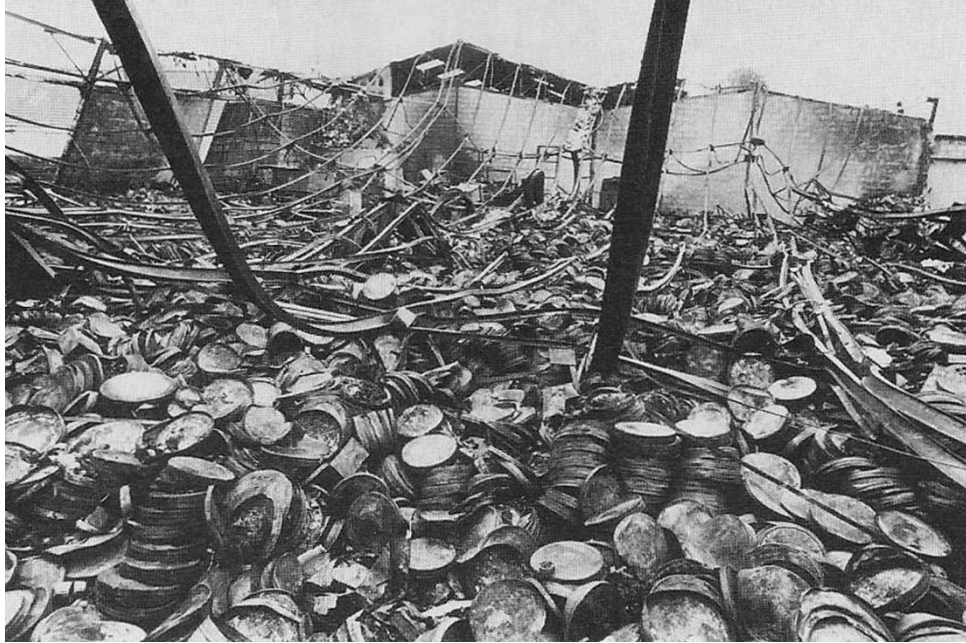
Nitrate vault fire
