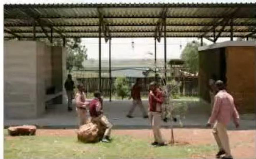
// Pokrit prostor za delo in učenje med učnico in sanitarijami // Covered space for work and learning between classroom and lavatories
