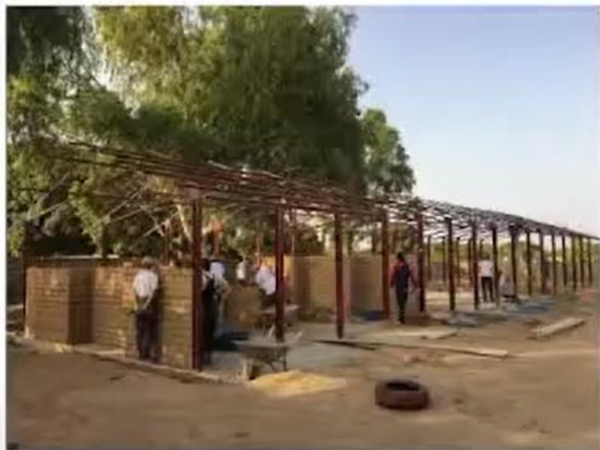
Źidanje cik-cak sten z namenom izboljšanja njihove stabilnosti Zig-zag bricklaying of the walls with the purpose of their stabilization
