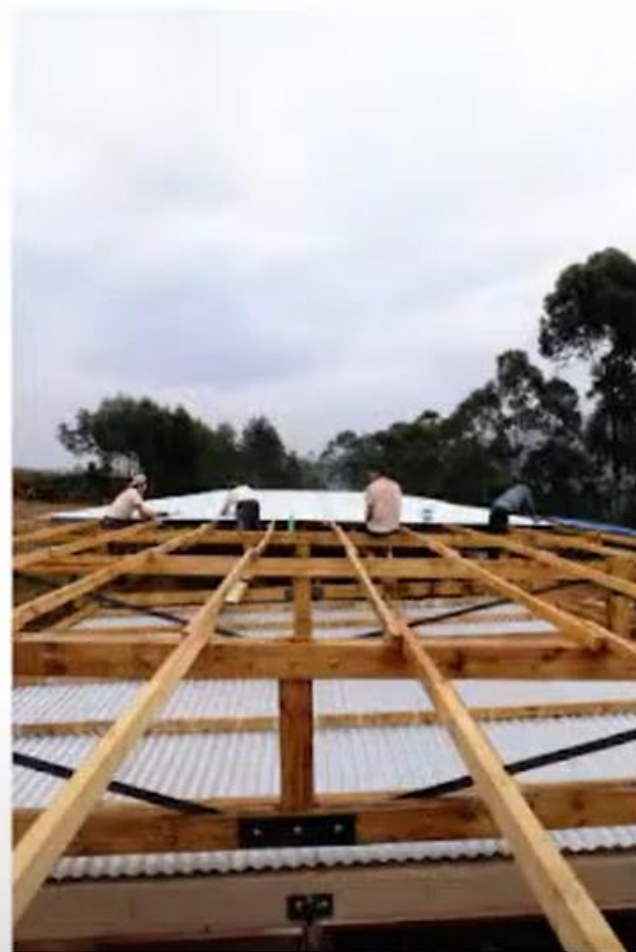
// Leseno ostrešje in dvojna streha, ki preprečuje pregrevanje notranjosti // Timber roof structure and double roof, which prevents the interior from overheating
