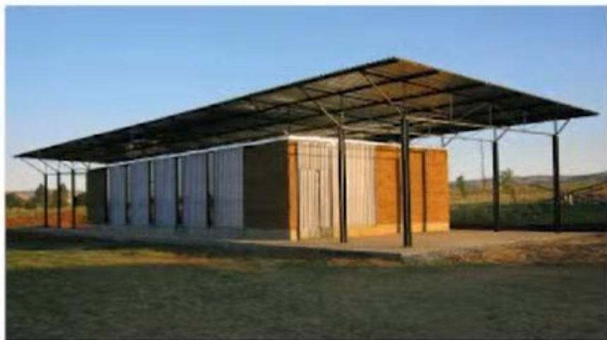
// Severna fasada s širokimi dvojnimi zasklenjvami in ozkimi okni // Northern facade with wide double glazing and narrow windows
