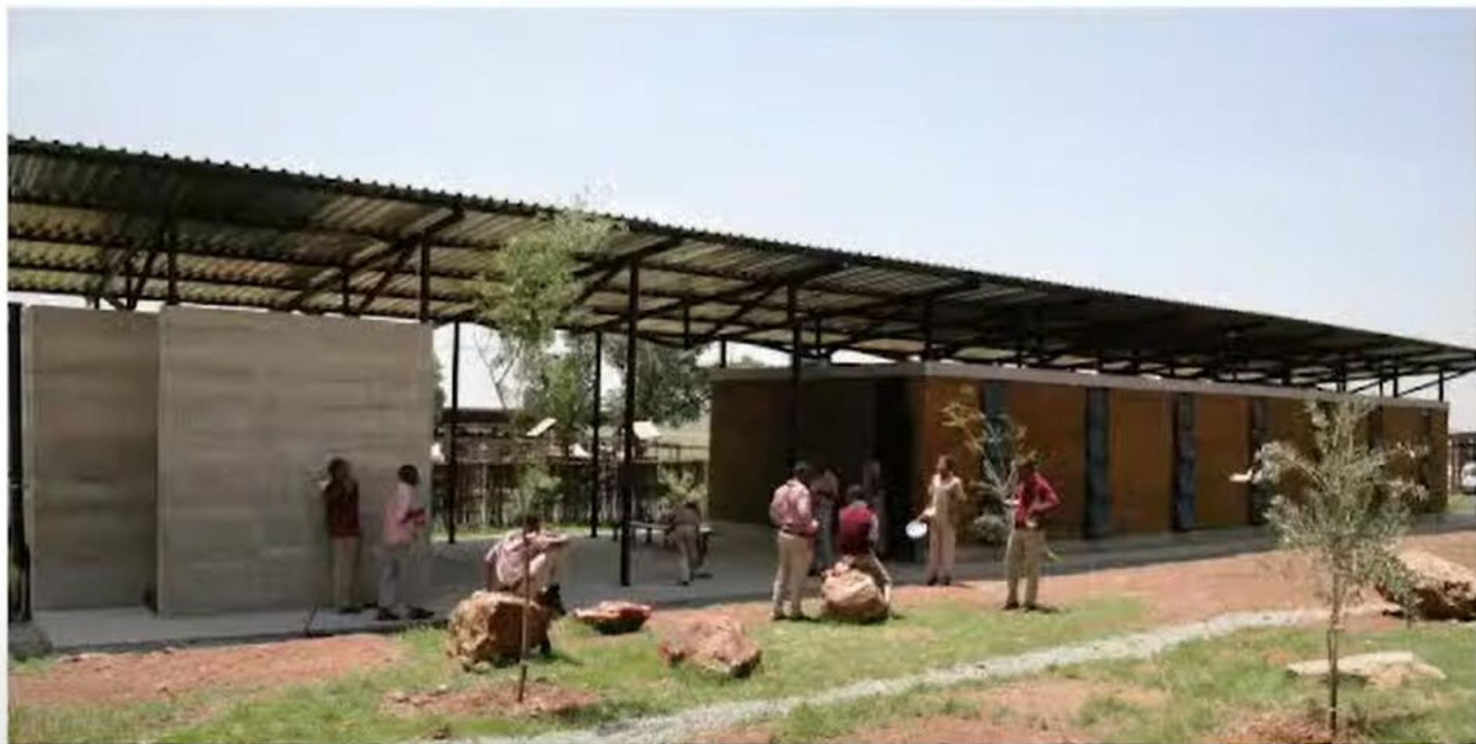
// Knjižnica in učilnica - večji in manjši kubi, ki ju prekriva lebdeča streha // Classroom and library - bigger and smaller cube, covered with a floating roof
