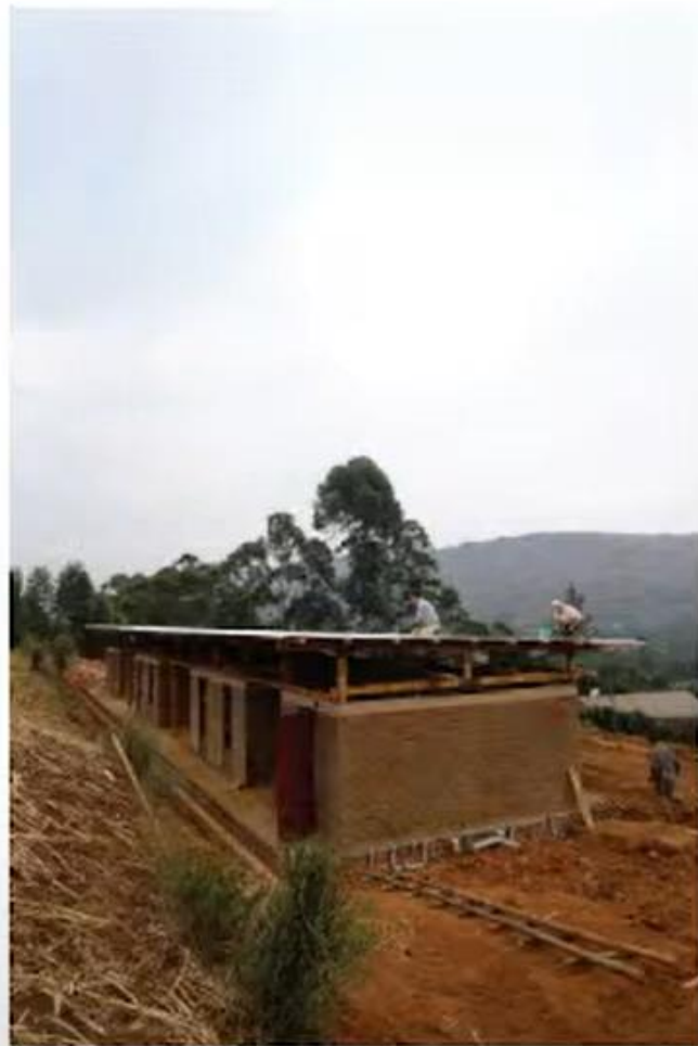
// Amasiko: tri hiške in med njimi odprti prostori, pokriti z lebdečo streho // Amasiko: three small houses and spaces in-between, covered with a floating roof
