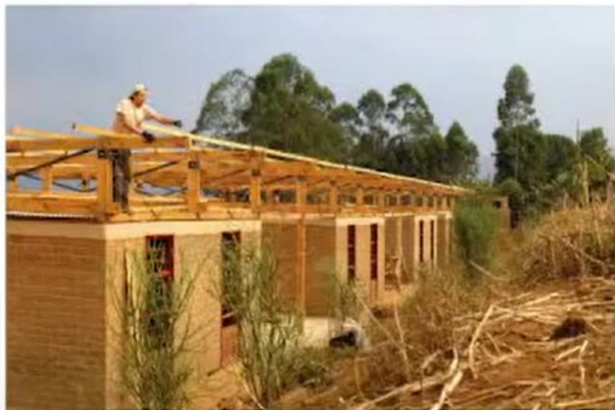
// Leseno ostrešje in dvojna streha, ki preprečuje pregrevanje notranjosti // Timber roof structure and double roof, which prevents the interior from overheating
