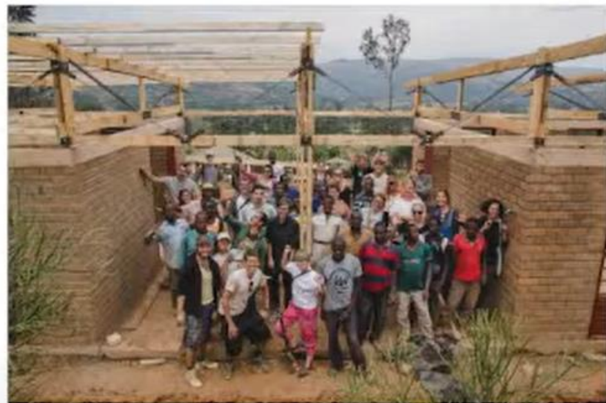
// Ekipa ob gradnji Amesko // Team at the construction of Amesko
