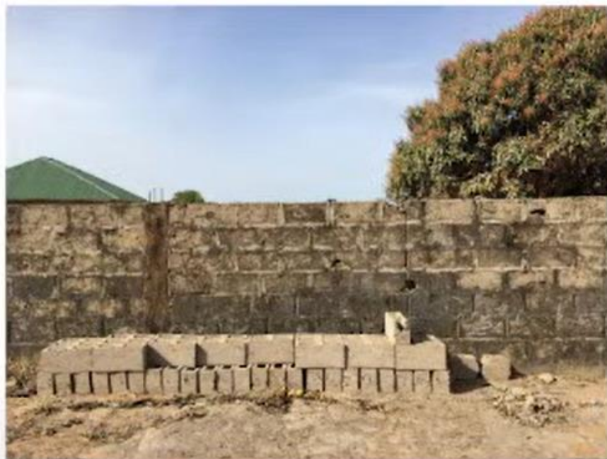
// Običajno gradivo: cementni zidaki, ki jih ljudje pogosto izdelajo sami // Common building material: cement bricks, often "home made"
