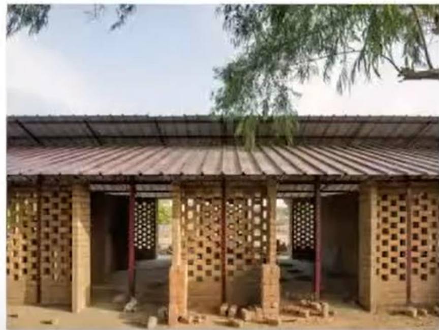
Ź Pravo kotni zaključki stabilizirajo stene in ustvarijo niše za klopi Perpendicular parts of the walls stabilize them and create niches for benches
