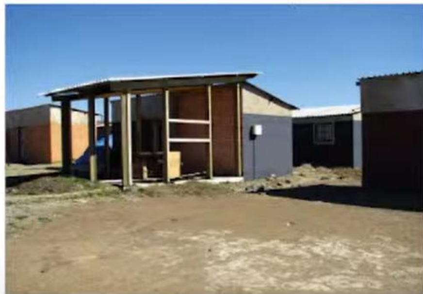
// Povečanje hiše enega od delavcev v townshipu: lesena konstrukcija, ki so ji sledila polnila iz butane slame in glin // Enlargement of the house of one of the workers in the township: wooden structure was later filled with rammed straw and clay
