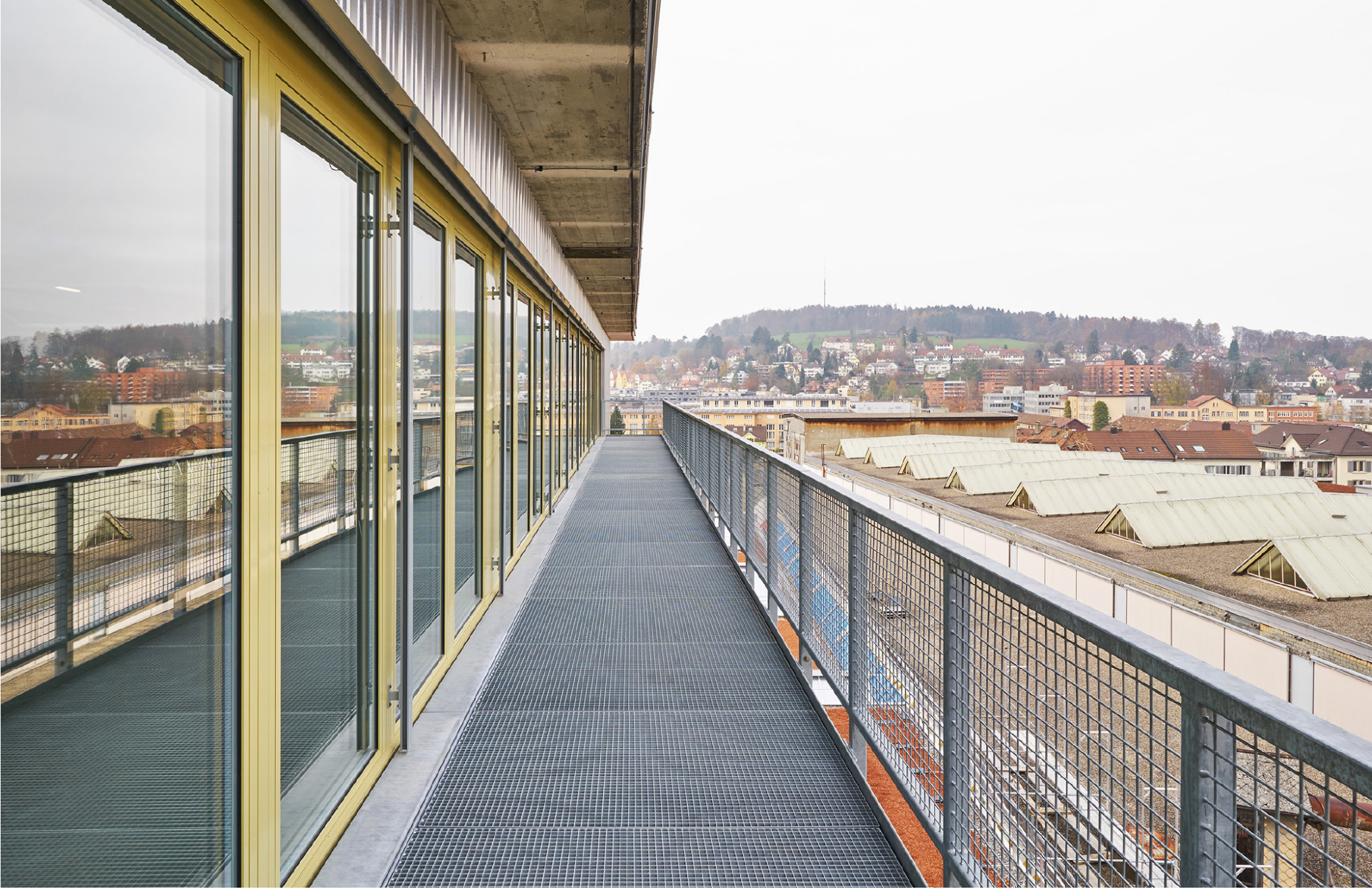
Halle 189 – Terrace to the city
