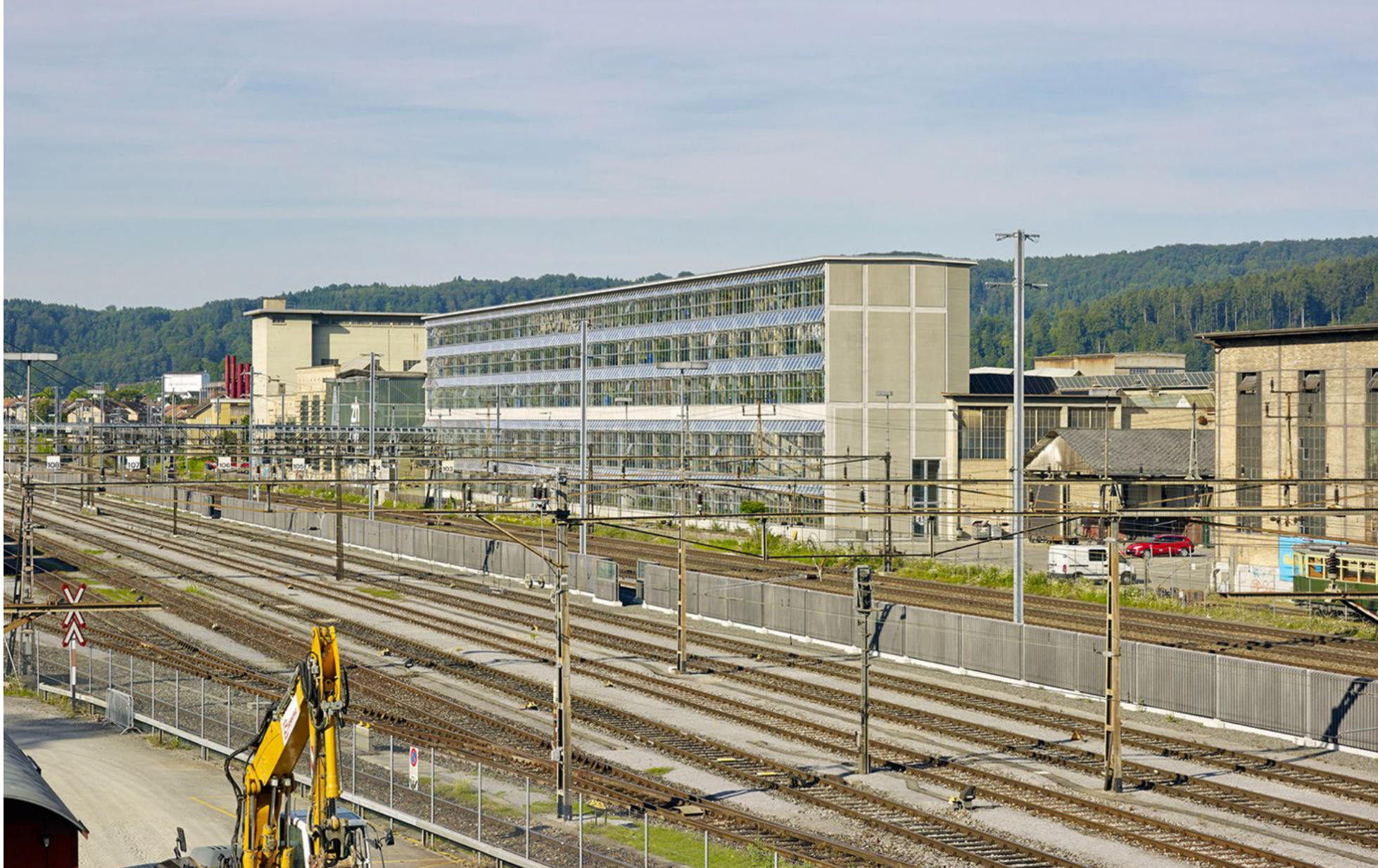
Halle 181 Vertical extension Kilga&Popp 2011-14
