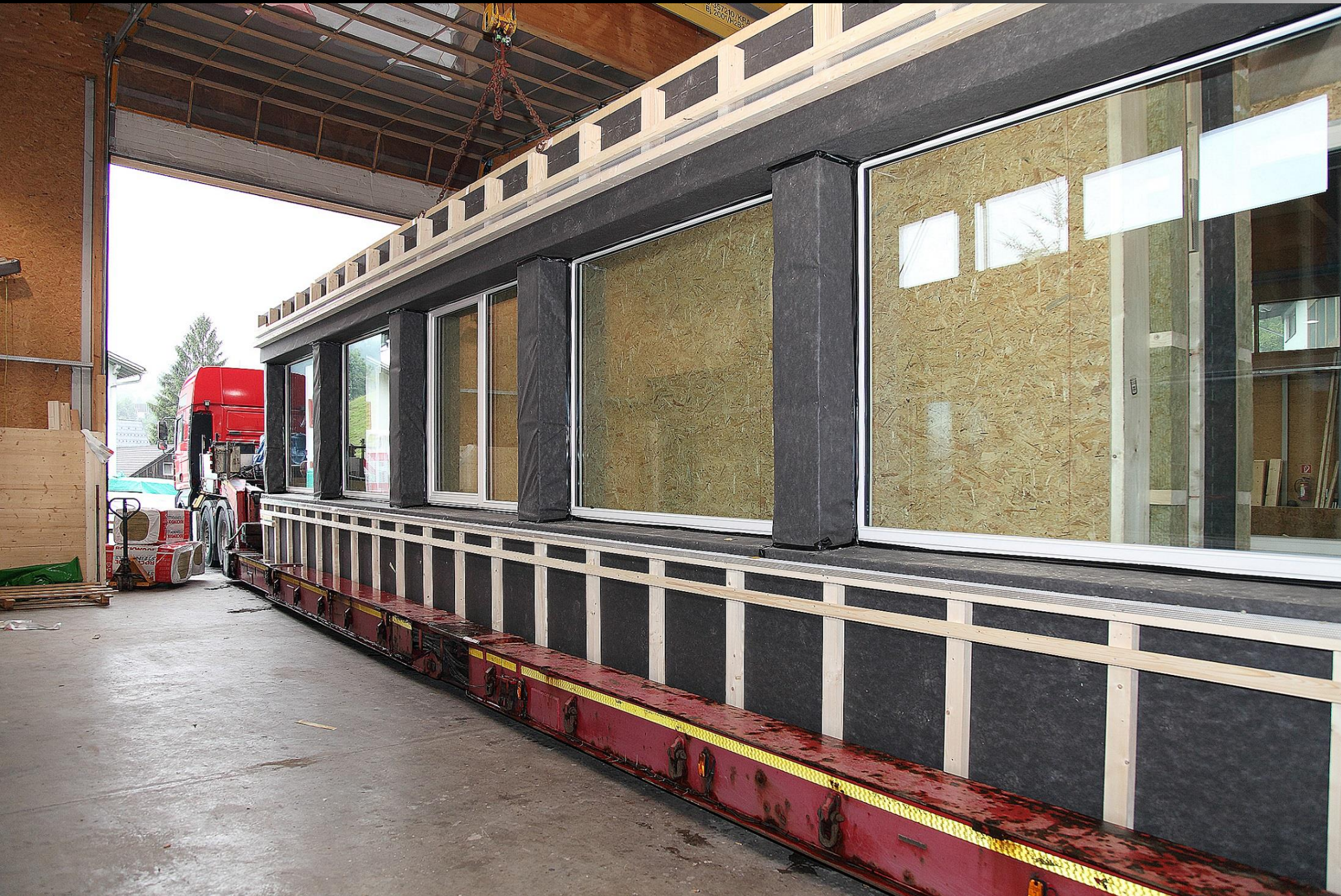
TRANSPORT PREFAB FACADE ELEMENT
