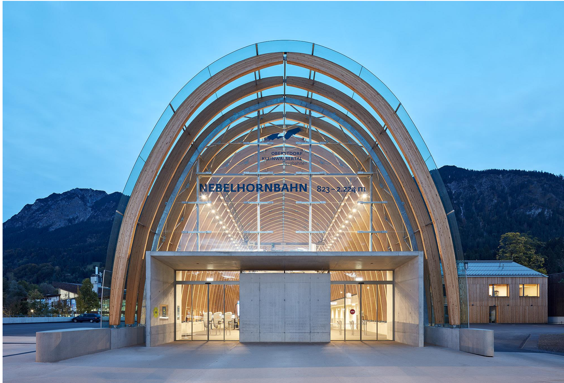
Nebelhorn ropeway station, Germany | Oberstdorf, HK Architekten
