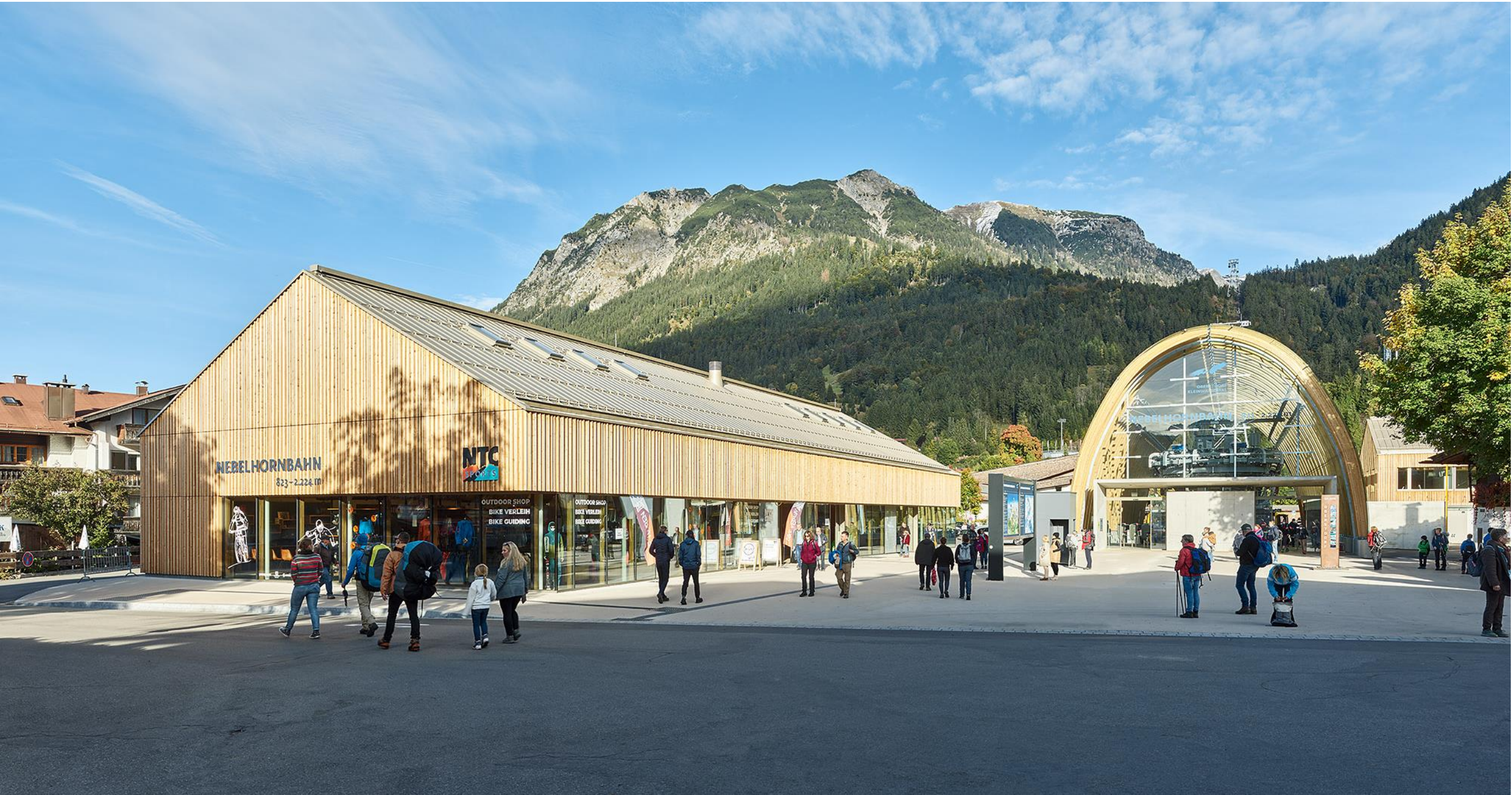
Nebelhorn ropeway station, Germany | Oberstdorf, HK Architekten
