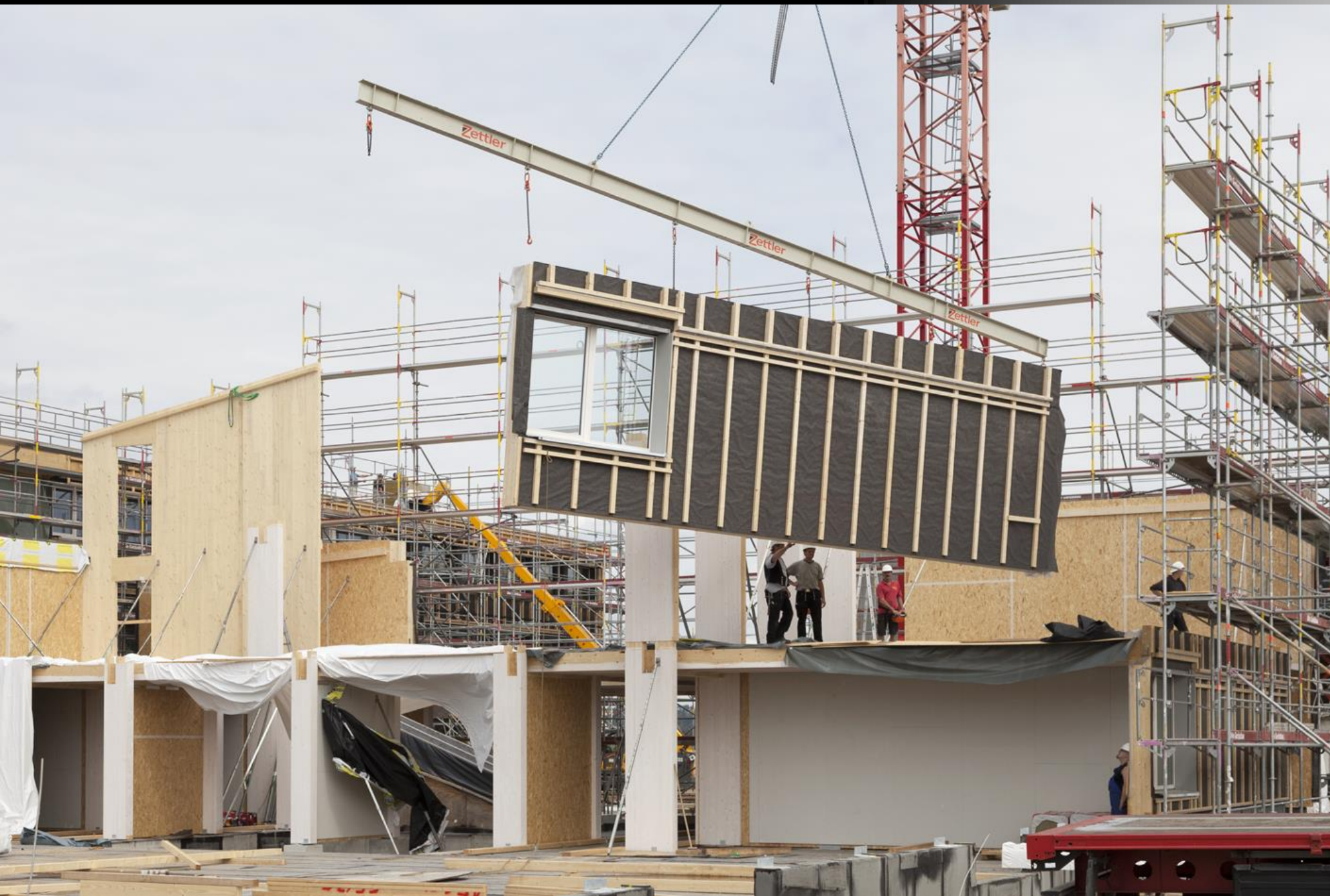
SITE ASSEMBLY PREFAB FACADE ELEMENT
