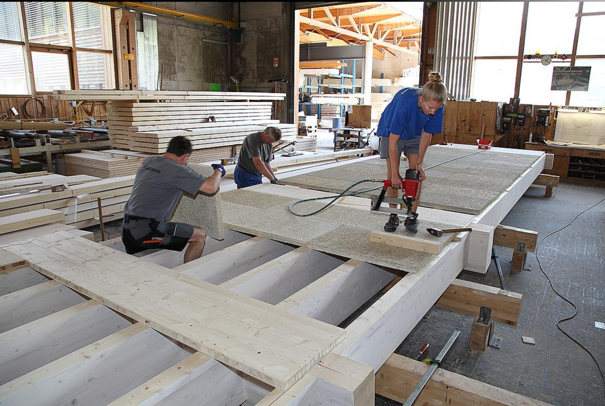
PREFABRICATION ROOF ELEMENT
