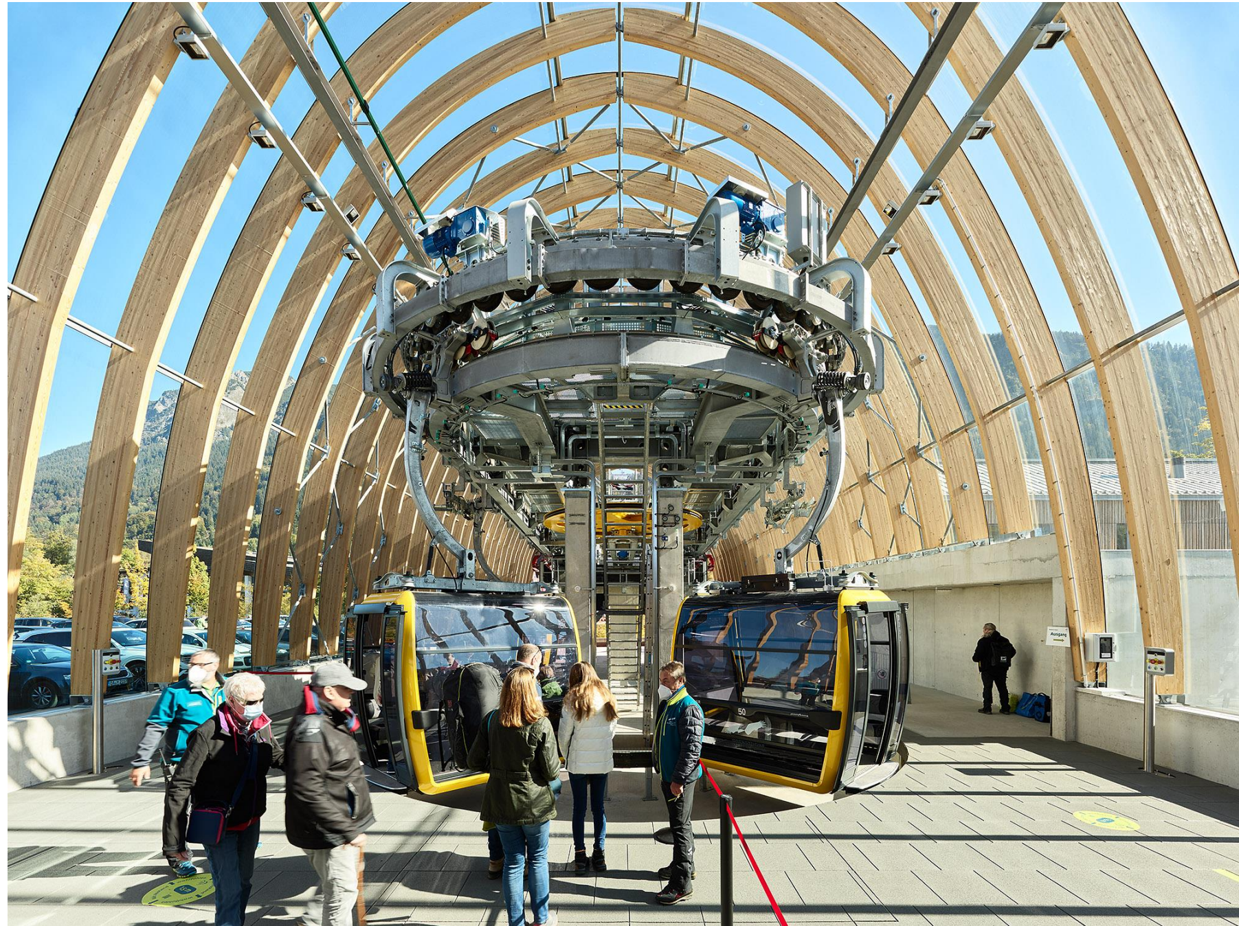
Nebelhorn ropeway station, Germany | Oberstdorf, HK Architekten
