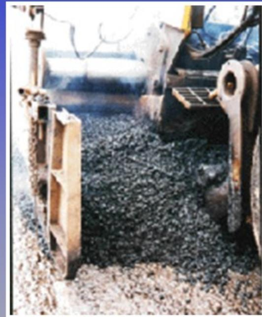
NEW: Lower noise, lower spray, use for thin resurfacing/regulating, Less rutting(?), Single Stage Installation = less delay
