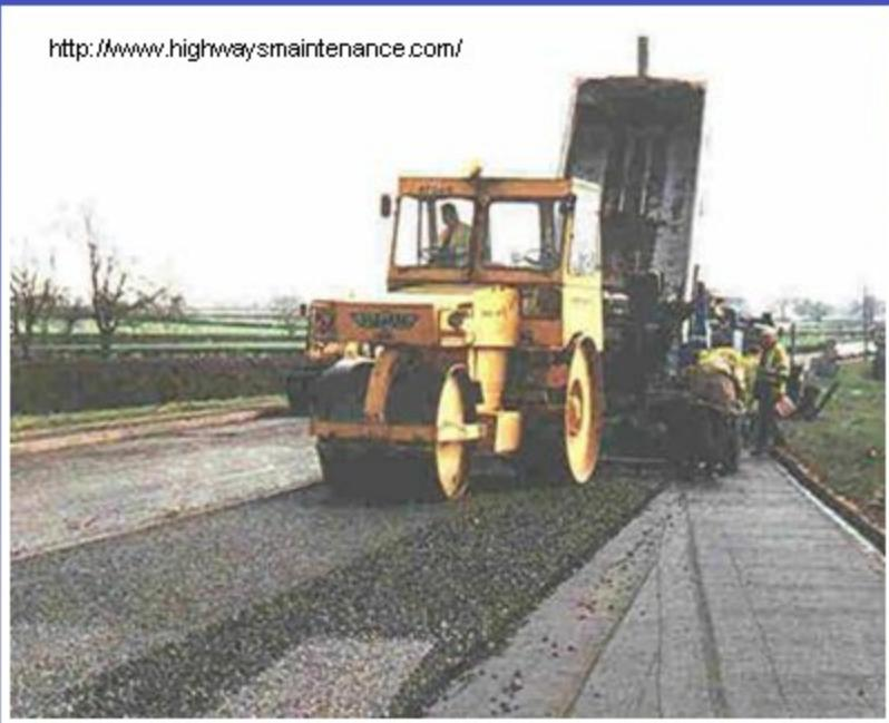
OLD: roadwork delays, perceived rutting problem, noise and spray issues. Two Part Installation
