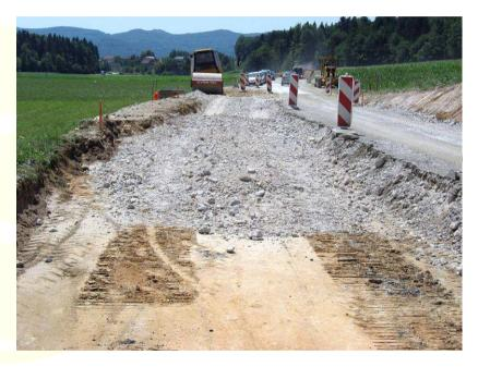
Determination of long term behaviour (bearing capacity, deterioration) of the unbound layer
