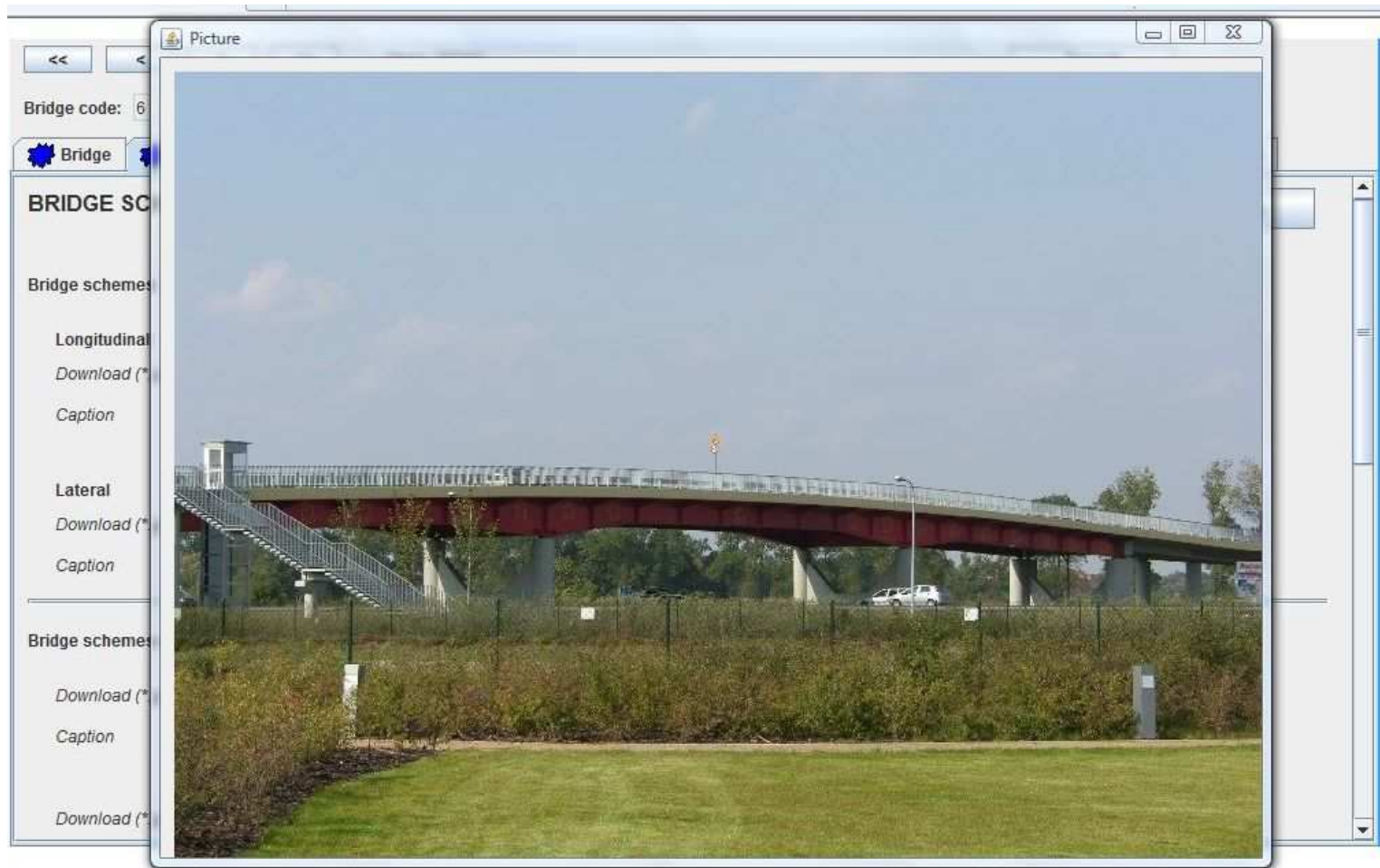
The photo of the bridge
