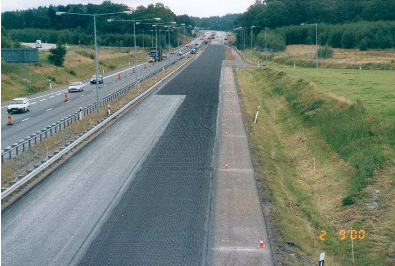
Steel reinforced test sections
