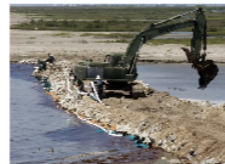
Workers build a land bridge
