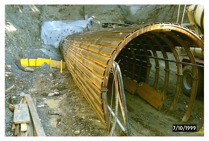
Shotcret of the surface; construction of "open air" steel support)
