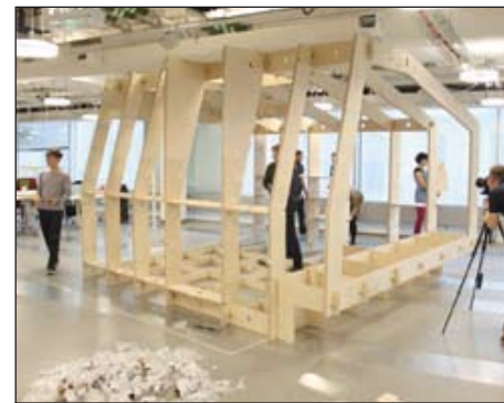
WikiHouse for the LDN Prototype Lab being assembled at Hub Westminster
